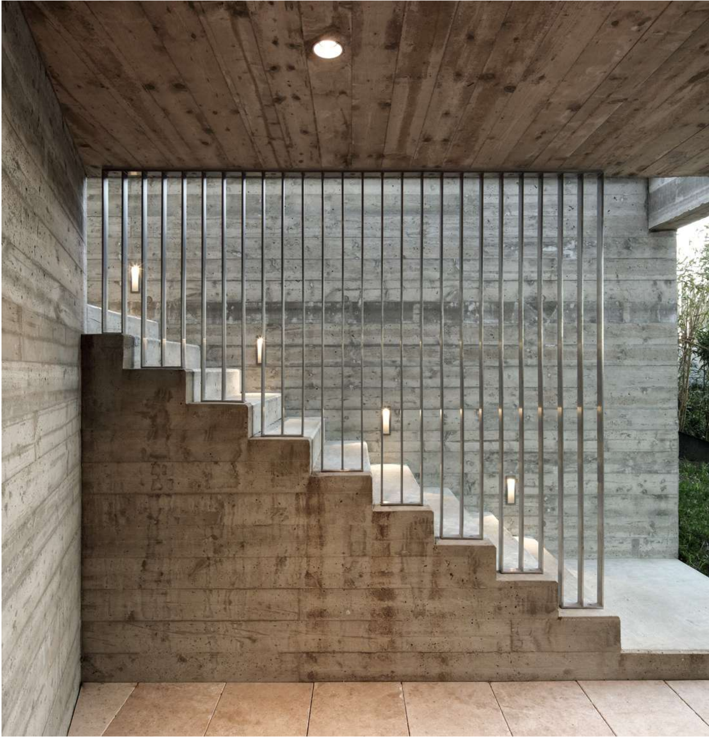
PRIVATE RESIDENCE | SPADO ARCHITECTS AUSTRIA
